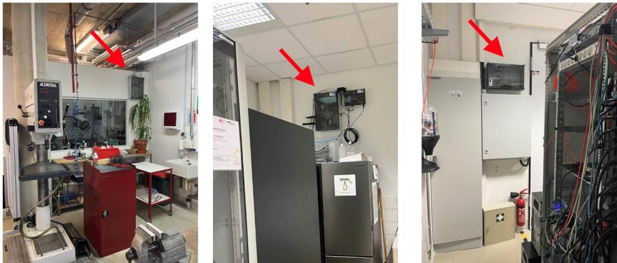
Figure 3.2 5G-enabled energy measurement in energy testbed. Mechanical workshop (left), electronics lab (center) and server room (right).
