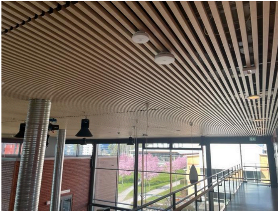
Figure 141: Example of 4G/5G Ericsson radio dots forming the CARL-W testbed and providing non-public connectivity at Karlstad University.
