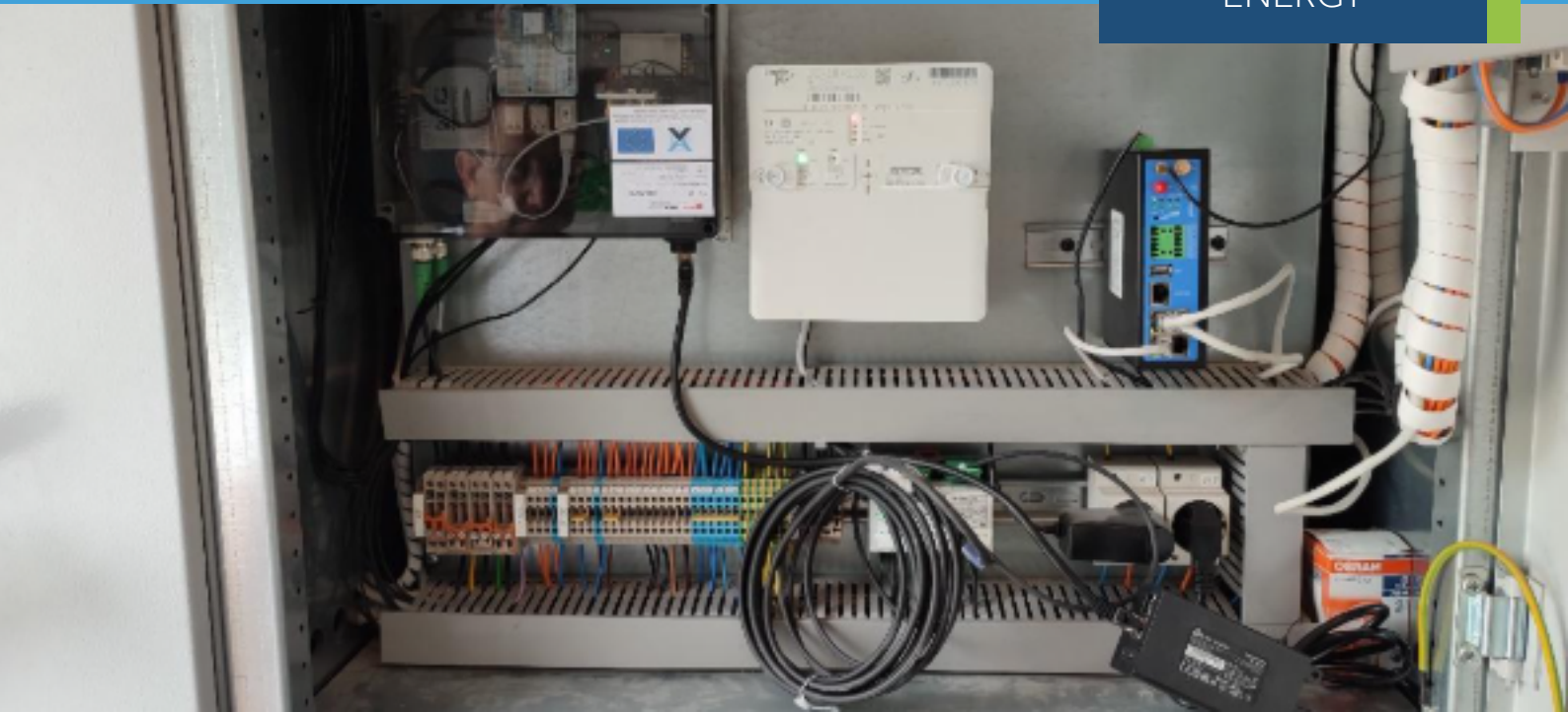
Figure 180: Installation of the edgePMU device in parallel with existing metering devices.
