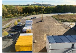
5G for construction
