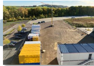
5G for construction
