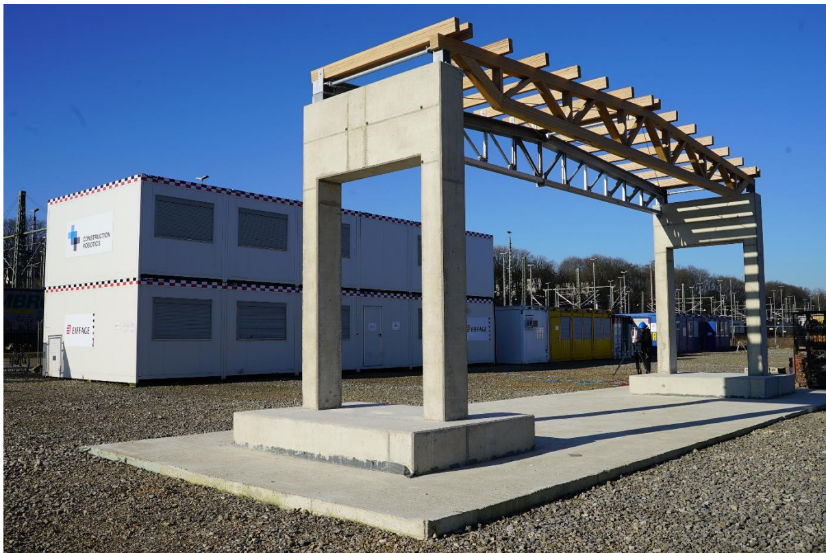
Figure 2.4 Example of a Demonstrator structure of the BMBF funded Project “Internet of Construction” at the previous testbed at RWTH Aachen Campus West [13].
