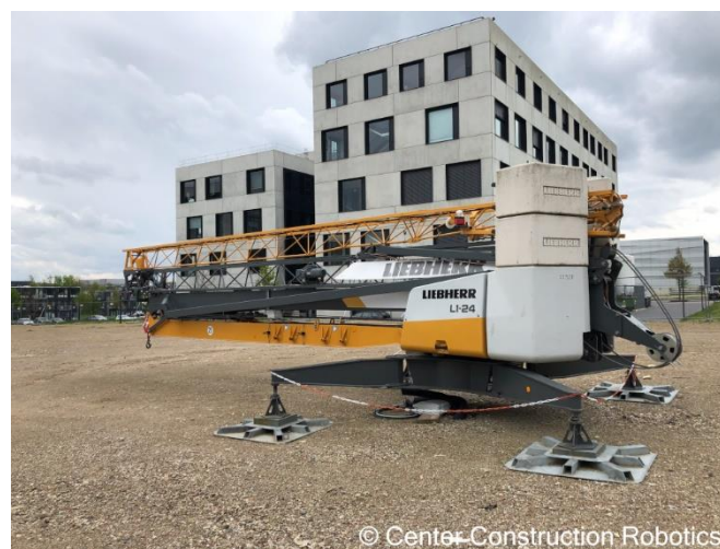
Figure 2: Tower crane at the Reference Construction Site (in folded state)
